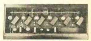
coupled, one stage of Samson impedance coupled, and the new Samson pushpull impedance stage. This combination gives a tone range and quality seldom heard. With the advent of the power tube there has been a tendency to ignore the push-pull method of amplification, which has long been considered superior to the single-tube per stage type. Sheldon's output stage uses two power tubes in the push-pull connection, and hence, is capable of tremendous volume without distortion.
